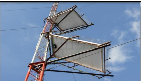
Fig 9 :Solar power for the radios of Wi-Fi tower with theft prevention measures in the forest region of Rajaborari, Madhya Pradesh
